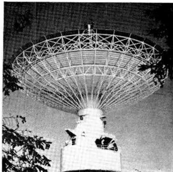
150 ft radio telescope of the National Research Council of Canada at Algonquin Radio Observatory, Lake Traverse, Ontario. The electronics system for controlling the steerable paraboloid was supplied by A.E.I. Electronics. The company's film "The Radio Sky", telling the story of radio astronomy, can be borrowed from A.E.I., 35 Grosvenor Place, London, S.W.1.
